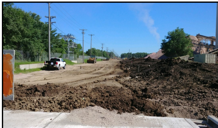
Louise Ave construction.
