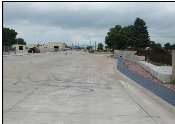
Madison Street wall construction.
