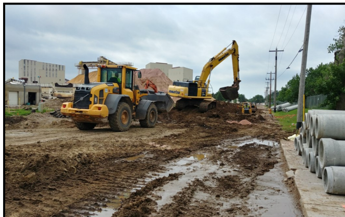
Louise Avenue utility construction.
