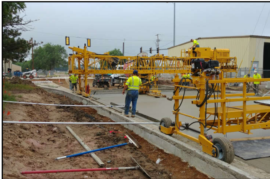
Placing Concrete Pavement at Madison Street and Louise Avenue Intersection.
