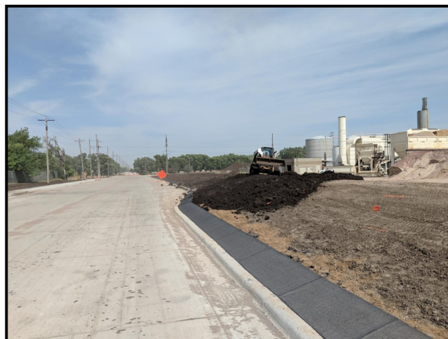
Placing topsoil behind back-of-curb along Louise Avenue
