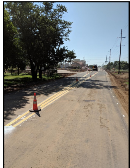
Pavement striping on north Louise Avenue
