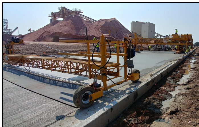
Louise Avenue Construction
