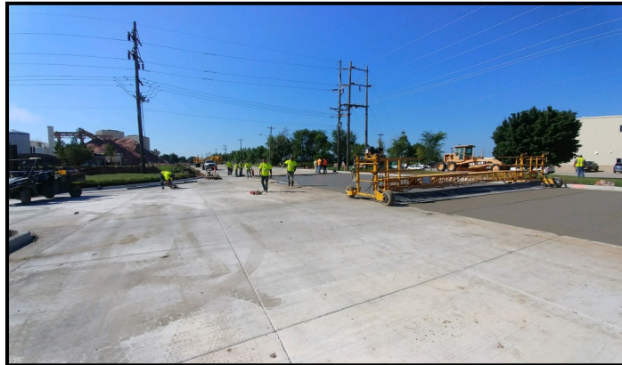
Louise Avenue Construction
