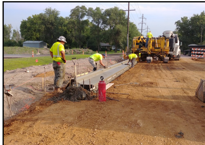
Louise Avenue Curb & Gutter Installation
