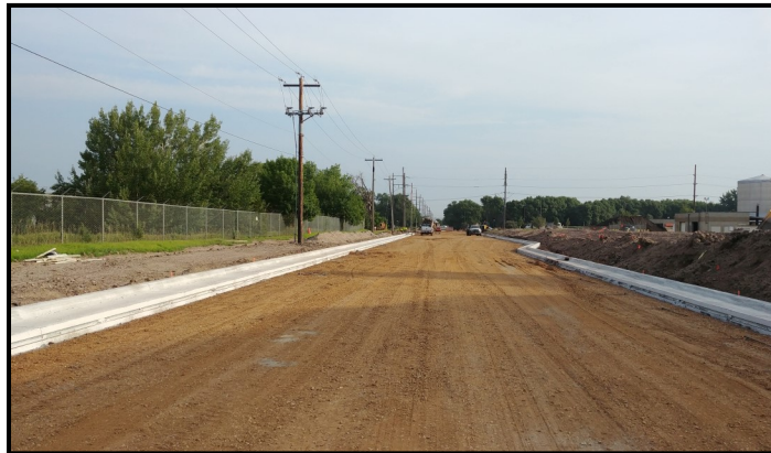
Louise Avenue Construction
