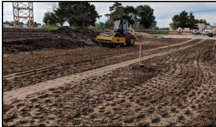
Louise Avenue construction
