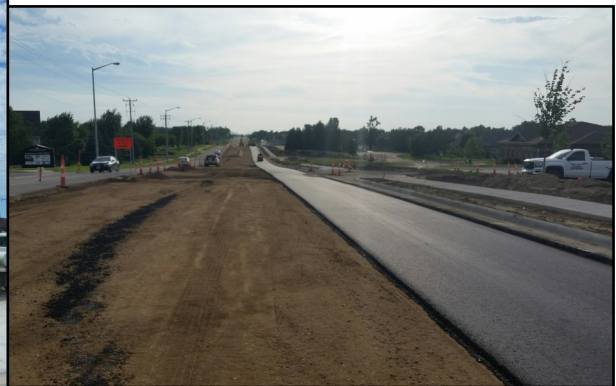
69th Street, looking west, with asphalt pavement placed on the gravel base during the asphalt paving operation
