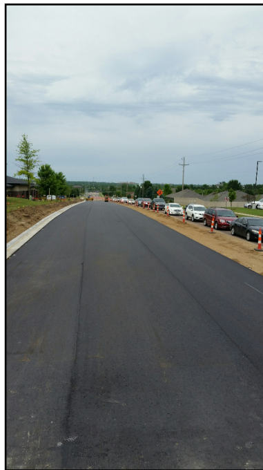
Western Avenue, looking north, with asphalt pavement on the southbound lanes.
